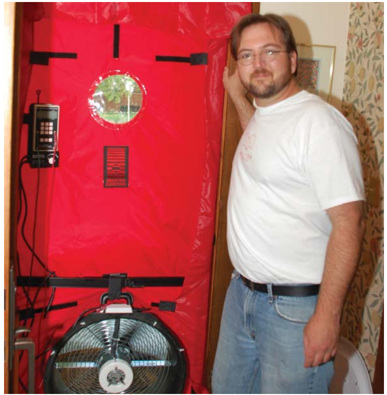
Steven Phoenix uses this 'blower door' to test homes for air leaks, which can be a major cause of heat loss and can also carry dust and pollutants from crawl-spaces and wall cavities inside.
